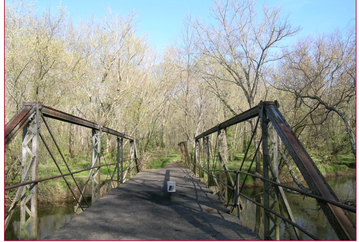
74B-012 Queen Anne Bridge Patuxent River at Queen Anne Bridge Road Queen Anne
