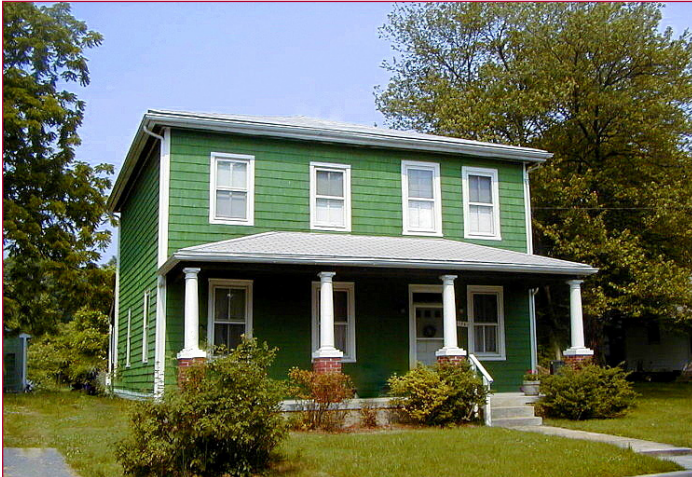
71B-002-08 Harmon-Phelps House 8706 Maple Avenue Bowie
