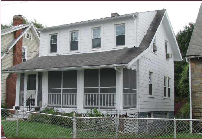
68-061-22 Quander-Dock House 4033 Webster Street North Brentwood
